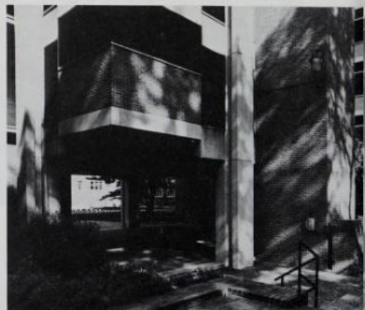
Entrance to the biology building. The concrete columns and cantilevered beams are precast.
