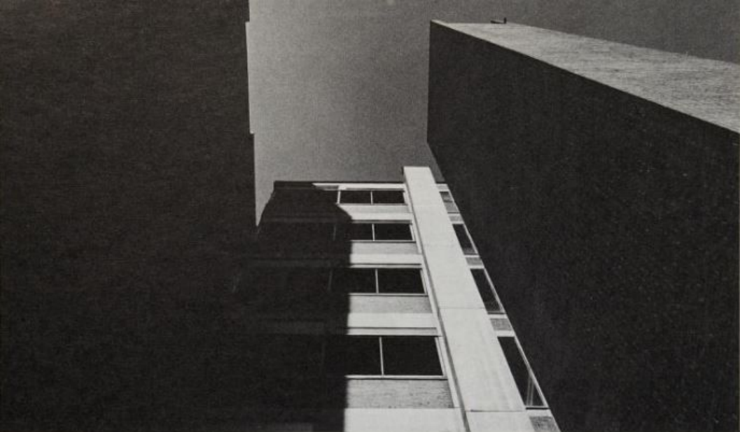
At the center are the laboratory floors. To the right is a stair tower. To the left is the main service core of the building.
