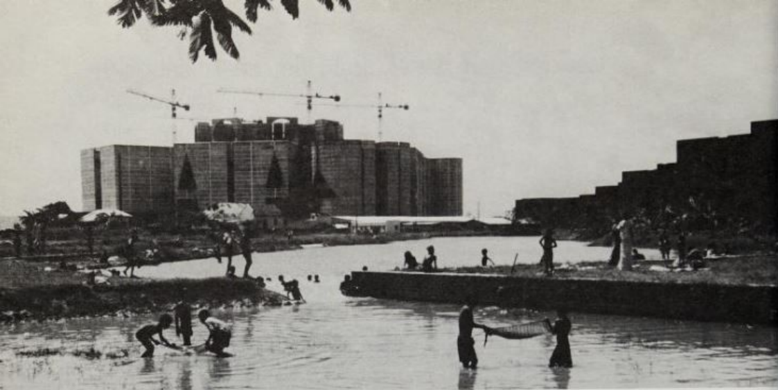
The National Assembly Hall seen from the Northwest. Cranes above the building are being used in construction.
